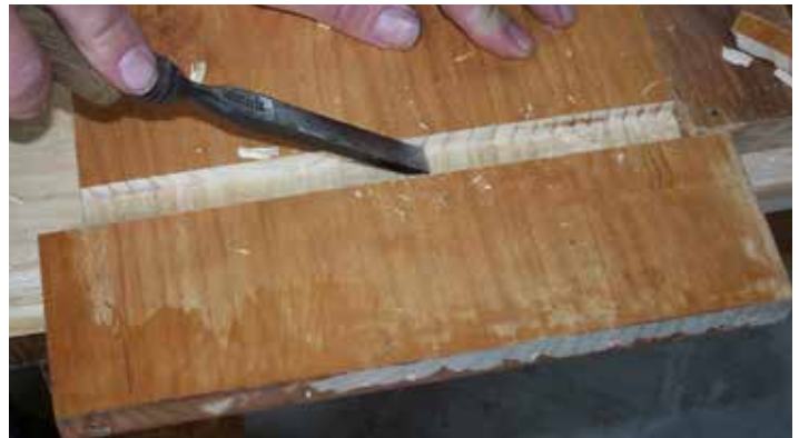
On more period accurate chests, the rebated joint for the base board may include a mortise for a tenon on the base board.
