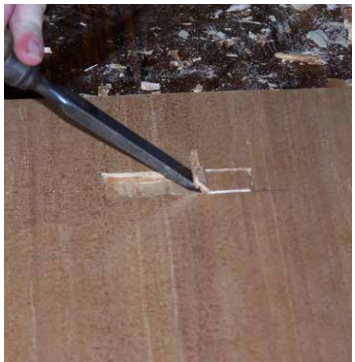
On more period accurate chests, the rebated joint for the base board may include a mortise for a tenon on the base board.
