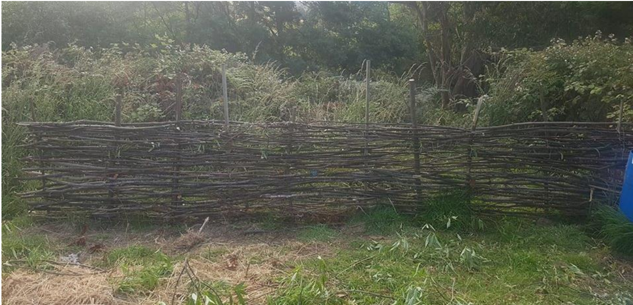
5m x 1m of fencing – approximately 15-16 hours of work
